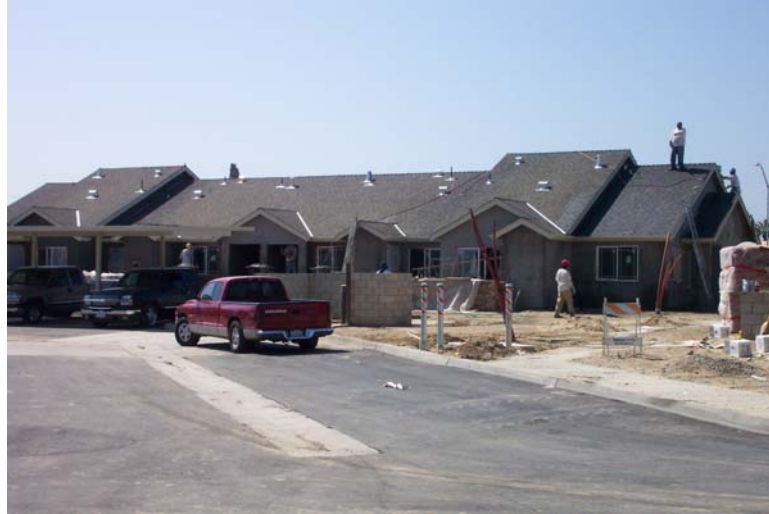
Biola Village Multifamily Project – 99% complete
