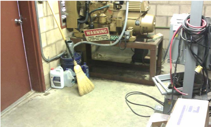
Transfer Switch 1" Conduit with Flex connecting to existing Generator. To be replaced as part of the project.
