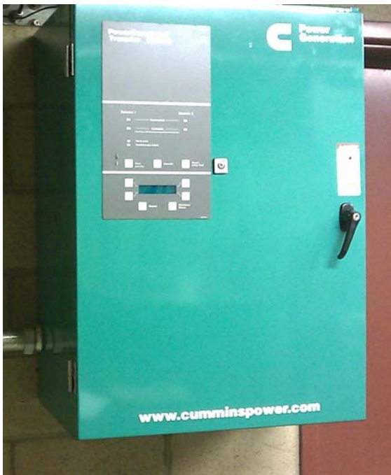
New Transfer Switch Installed October 2012 Model Number OTPC-10529809 SN A120296297
