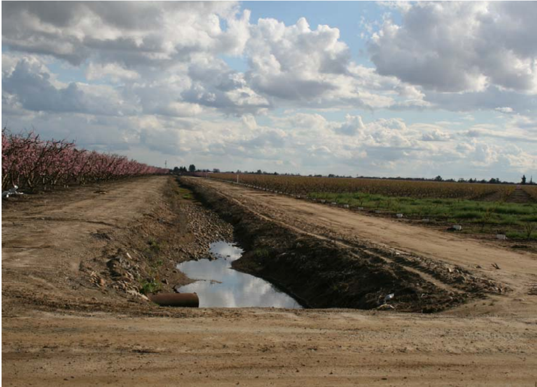
Fink Ditch water distribution canal.
