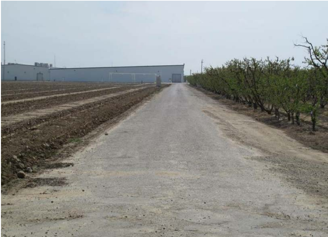
Fruit packing and shipping plant. View from Ranch Road facing South.
